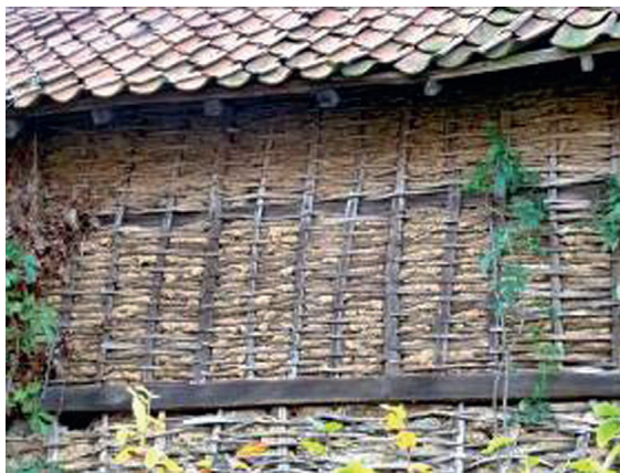
15 Op de Vink: oetgereëgend rijwerk in de vakke, 2014.
